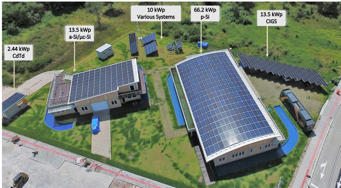
Figure 1. PV systems at Lab. Fotovoltaica-UFSC, Sapiens Parque.
