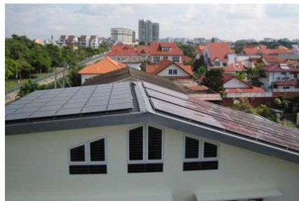
Figure 12- Residential PV system in Singapore. Metal roof and poor ventilation in the area make this site one with the highest k-values of systems under investigation.
