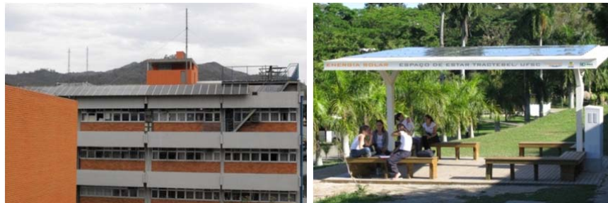
Figure 9- System BR1 (left) has been under operation for 14 years and it was the first grid-connected PV system in Brazil. It is installed at the Mechanical Engineering Department building of UFSC. System BR2 (right) is also located inside the UFSC campus in Florianópolis.
