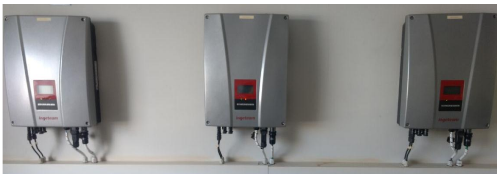
Figura 4 – Inversor INGETEAM modelo Ingecon Sun Lite 3,68TL
